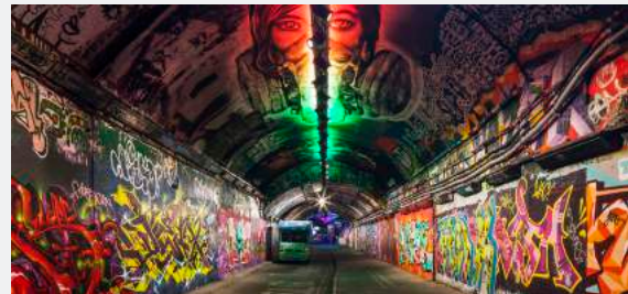
LEAKE STREET ARCHES, SE1 (25,000 SQ FT OF LEISURE)
