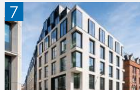
7 THE CURSOR BUILDING, CHANCERY LANE, WC2
