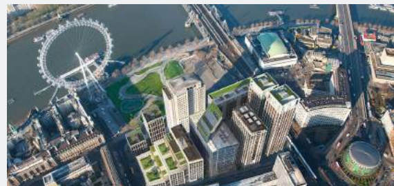
SOUTH BANK PLACE, SE1 (48,000 SQ FT OF RETAIL & LEISURE)
