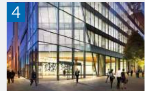
4 TWO SOUTHBANK PLACE, SE1
